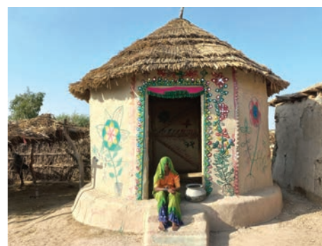
Fig. 8. Completed LOG shelter, Pono Colony, Mirpurkhas, Sindh, 2022.
