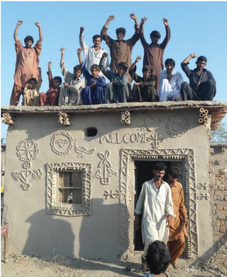
Fig. 1. Completed roof of a building sponsored by Lari Green Shelter (LGS) being tested for load-bearing capacity, Tandou Allahyar, Sindh, Pakistan, 2011. All images courtesy of the Heritage Foundation of Pakistan, unless otherwise noted.
