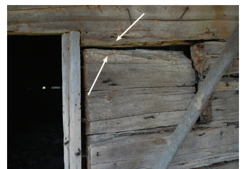
Fig. 5. Cole Barn, Clark County, Indiana, 1842, showing the eroded outer portion of exposed timbers, 2021. When the outermost rings are lost, the exact year of felling cannot be determined.
