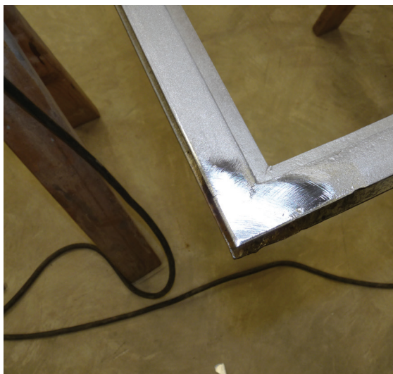
Fig. 3. Completed repair of severe corrosion by replacement of missing metal, 2011.
