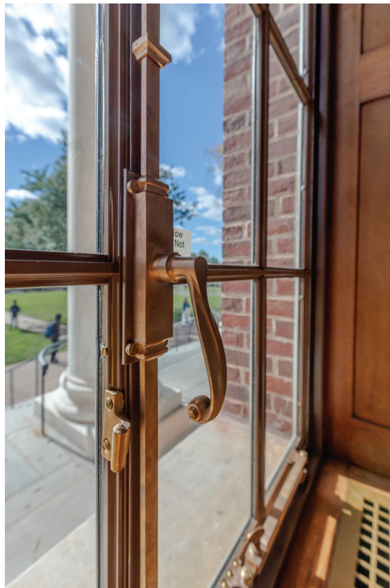
Fig. 5. Olin Library, Middletown, Connecticut, built 1928, showing a restored window handle made by breaking the bronze cremone operating handle down into its original 12 pieces, recasting the broken splines and worn operating arms, and refinishing the handle, 2018.
