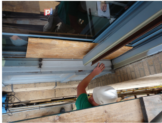
Fig. 4. Replacement subframe section tack-welded in position in situ, 2011.
