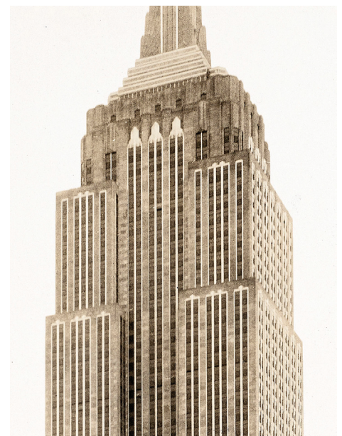
Fig. 4. Empire State Building, New York, New York, 1931, window assemblies showing the contrast between the bright chrome-nickel steel of the vertical trim and the dark windows and deplated spandrels. Empire State Building archive, 1930–1969, Avery Architectural & Fine Arts Library, Columbia University.
