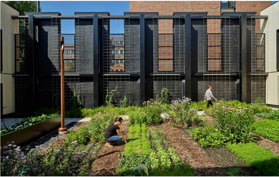
Fig. 3. Stanley Center for Peace and Security, courtyard created by selective removal of existing building volume to increase daylighting, reduce operational costs, and provide outdoor program space. Photograph by Integrated Studio, 2023.
