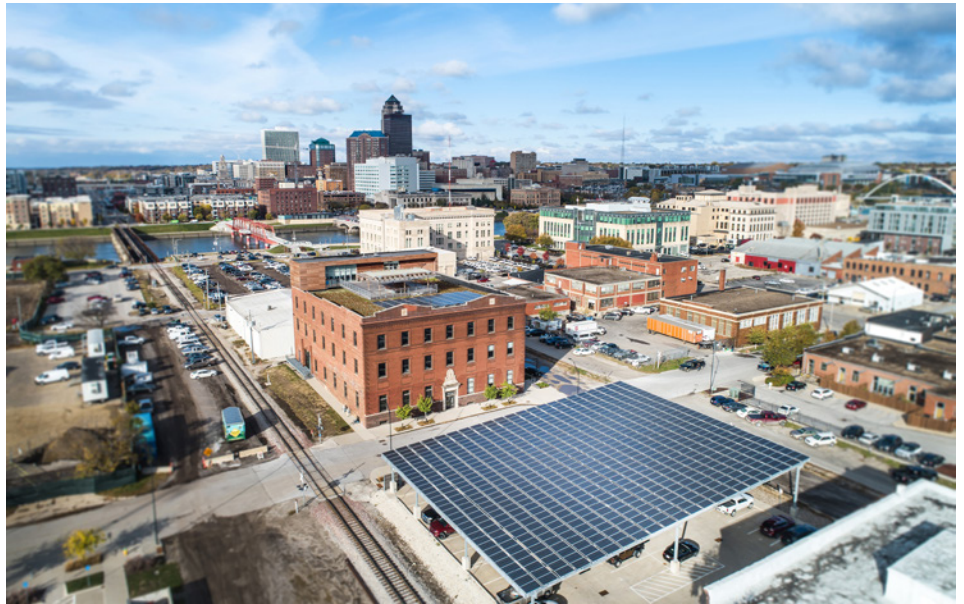
Fig. 8. Market One, solar photovoltaic panels located on the rooftop and car-park canopy across the street to preserve the historic structure's appearance while providing renewable energy. Photograph by Neumann Monson Architects, 2020.
