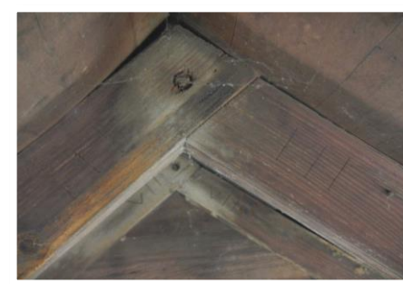
Figure 6: Trusses numbered with carved roman numerals.
