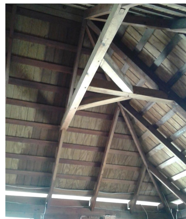
Figure 4: unique T-Truss in roof space hold the walls and roof together.
