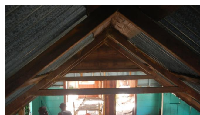
Figure 6: Trusses numbered with carved roman numerals.
