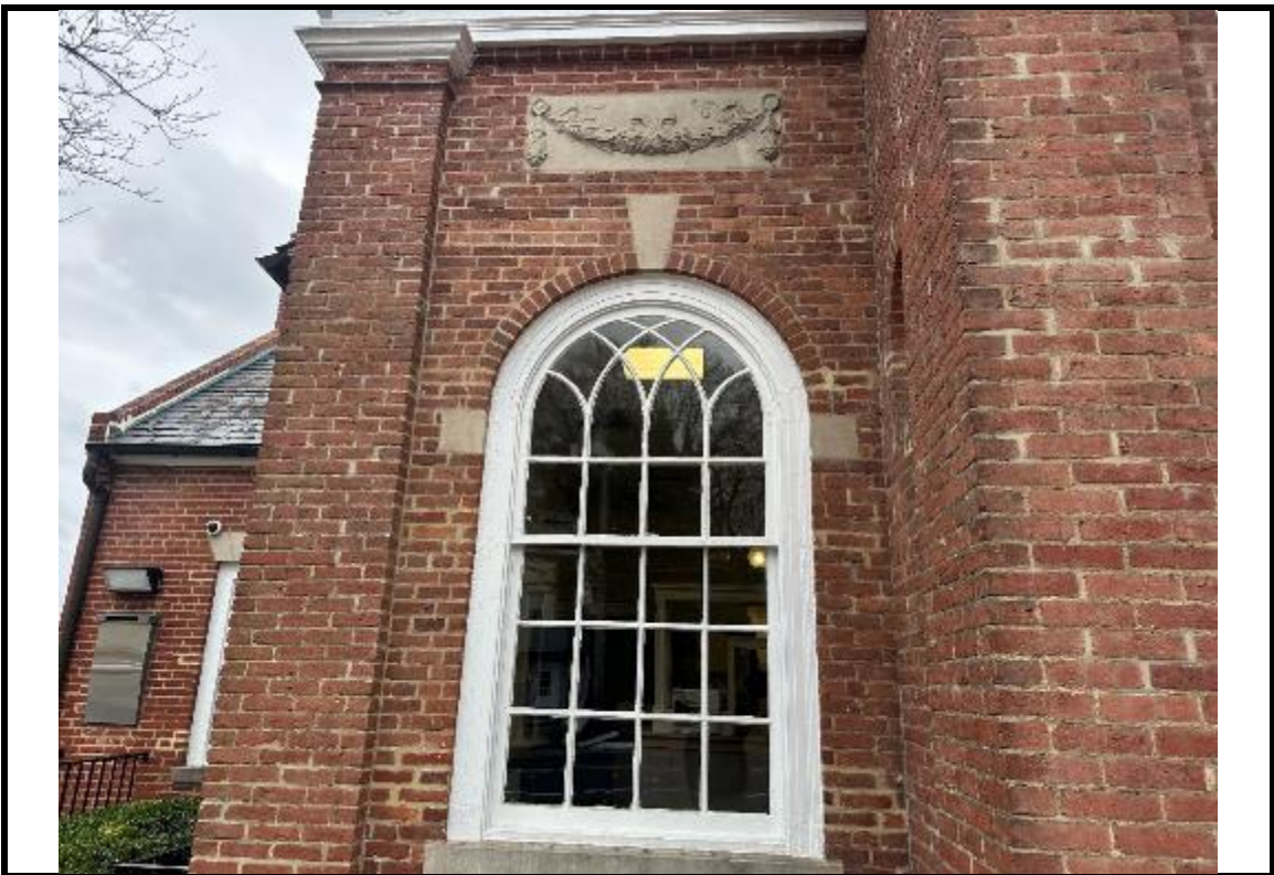
Photograph 24: Typical single-hung arched window.
