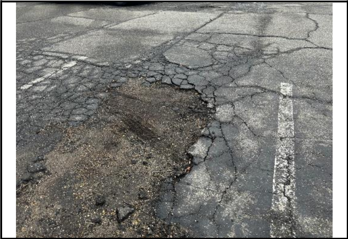
Photograph 9: Typical condition of asphalt pavement.
