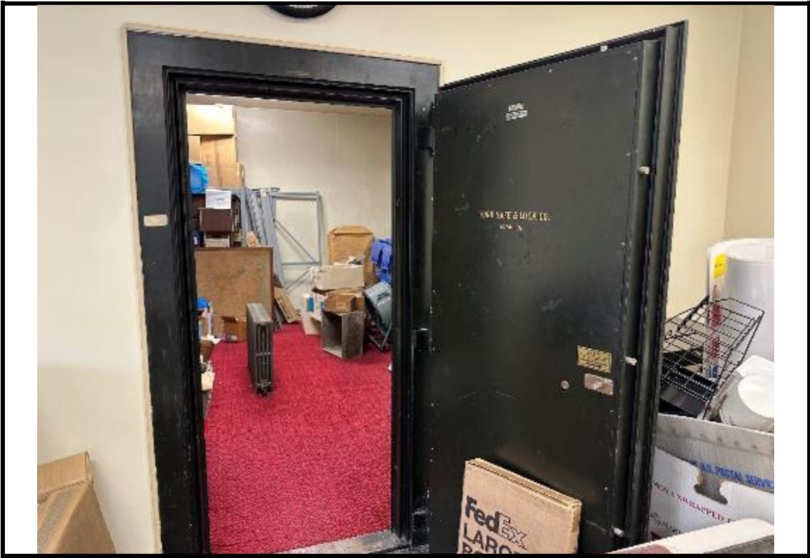
Photograph 47: Vaulted area safe door.
