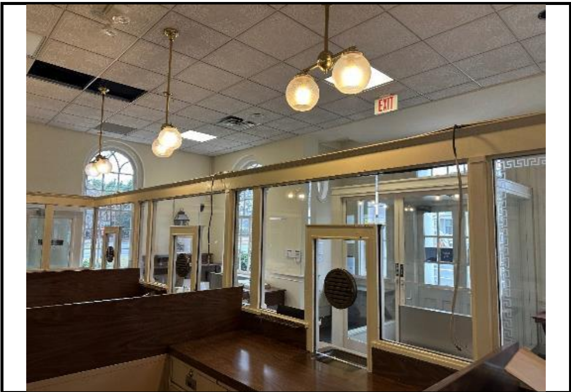
Photograph 42: Back view of bank teller stations.
