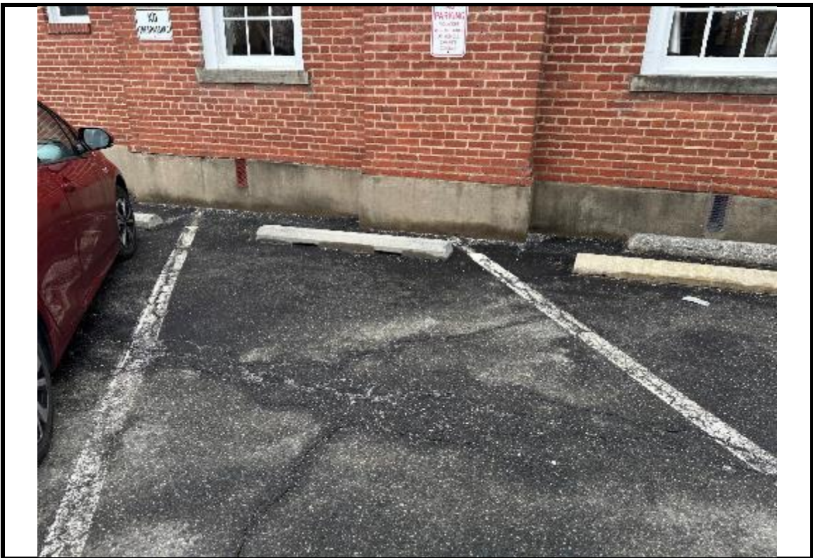
Photograph 6: Parking spaces adjacent to the building.
