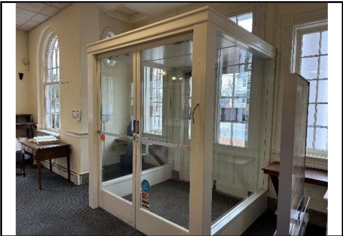
Photograph 40: Main entrance vestibule.
