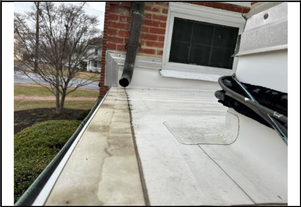
Photograph 35: Partial view of low TPO roof.
