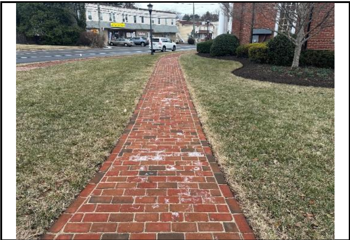
Photograph 12: Paver sidewalk along the north elevation.
