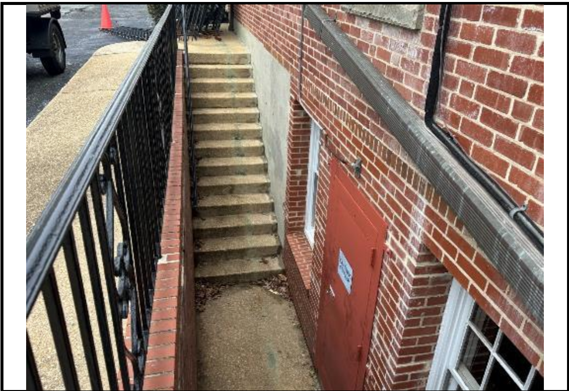
Photograph 16: Concrete stairs at the rear elevation for the basement egress.
