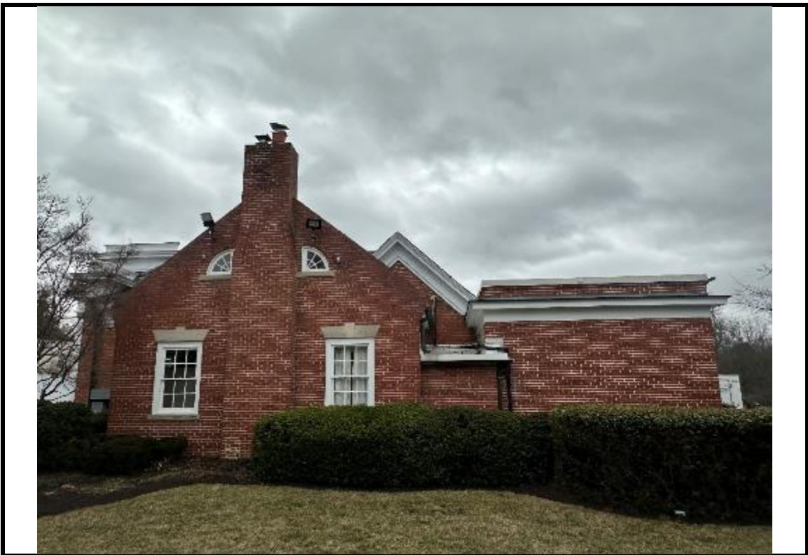
Photograph 22: General view of the east elevation.
