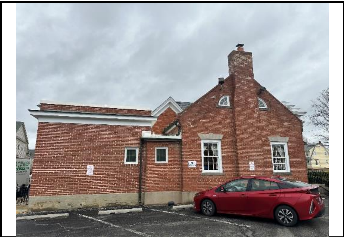
Photograph 20: General view of the west elevation.
