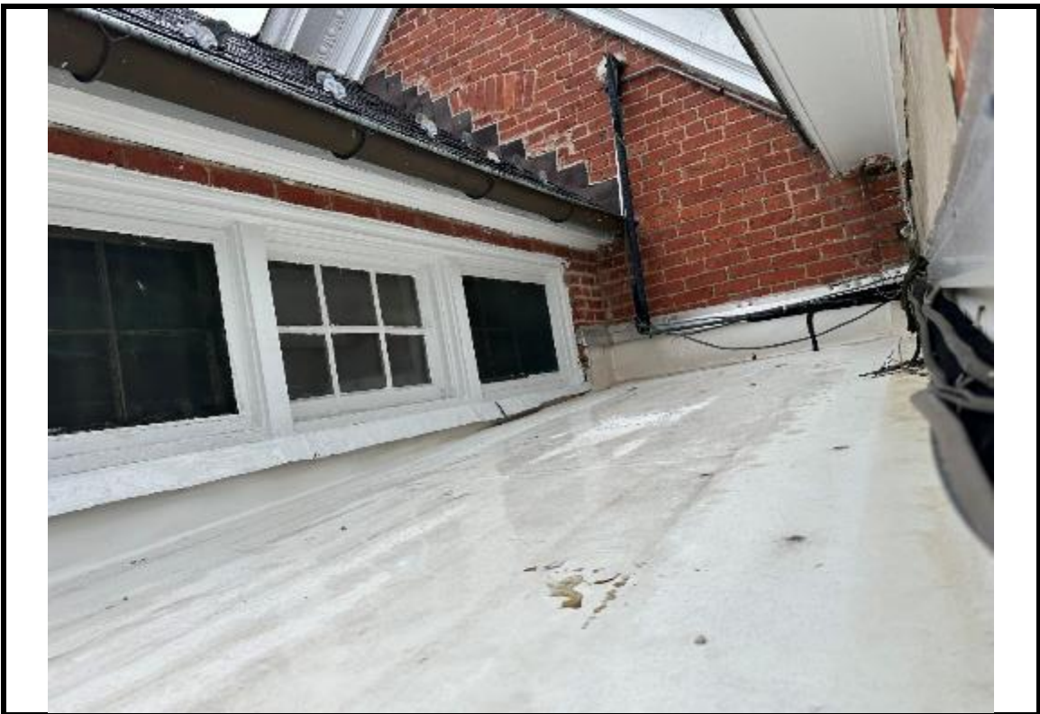
Photograph 36: Partial view of low TPO roof.
