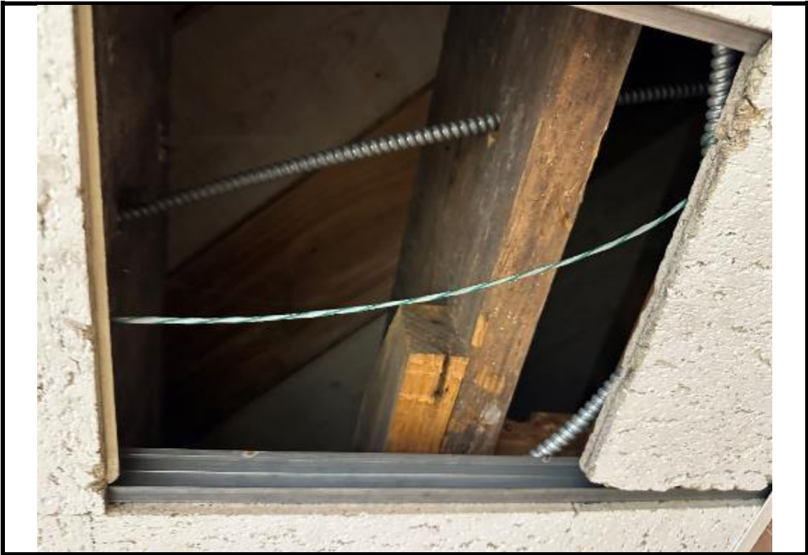
Photograph 53: Typical floor joist and 2x wood decking.
