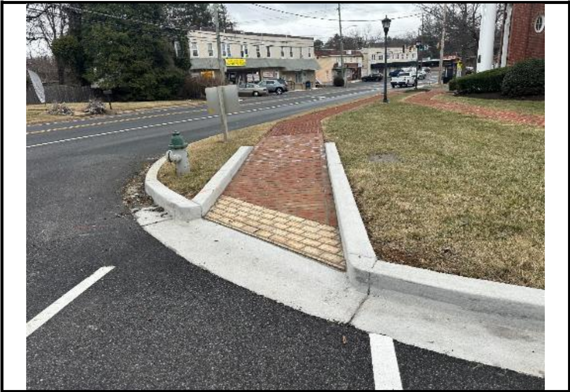
Photograph 11: Typical paver sidewalk along the public right of way.
