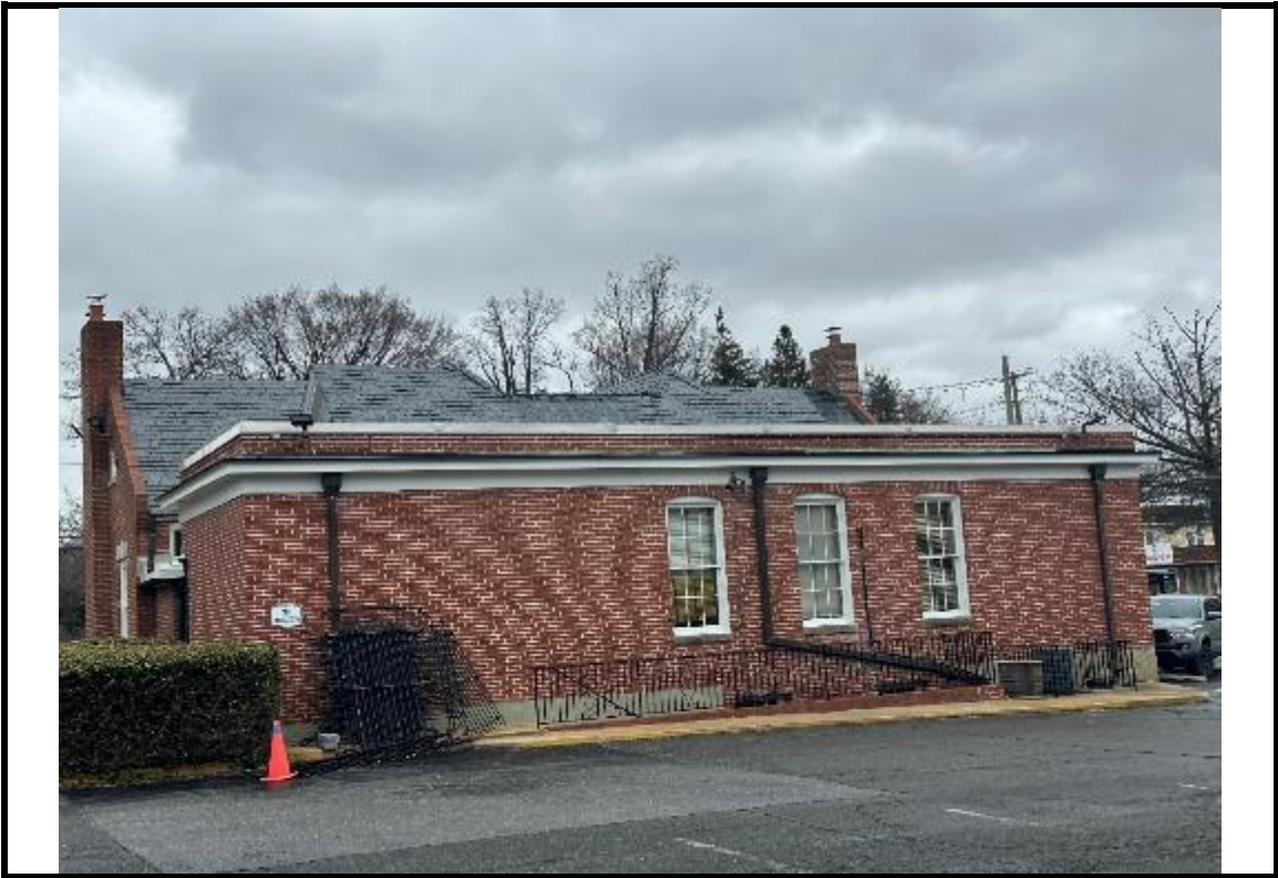
Photograph 21: General view of the south elevation.
