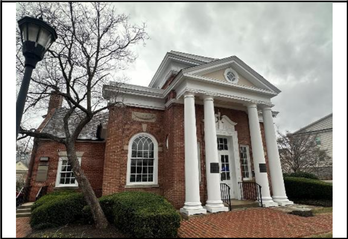
Photograph 1: Sandy Spring Bank general view of building.
