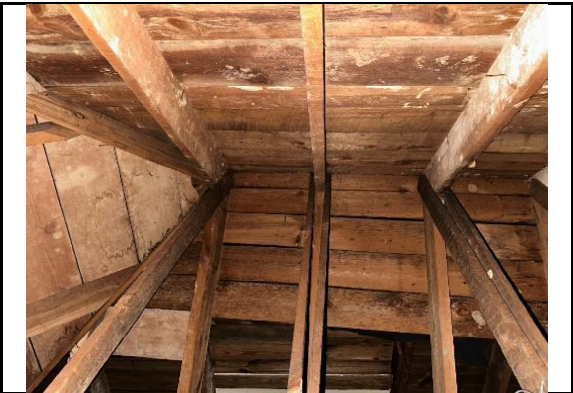
Photograph 54: Typical roof framing and 2x roof decking.
