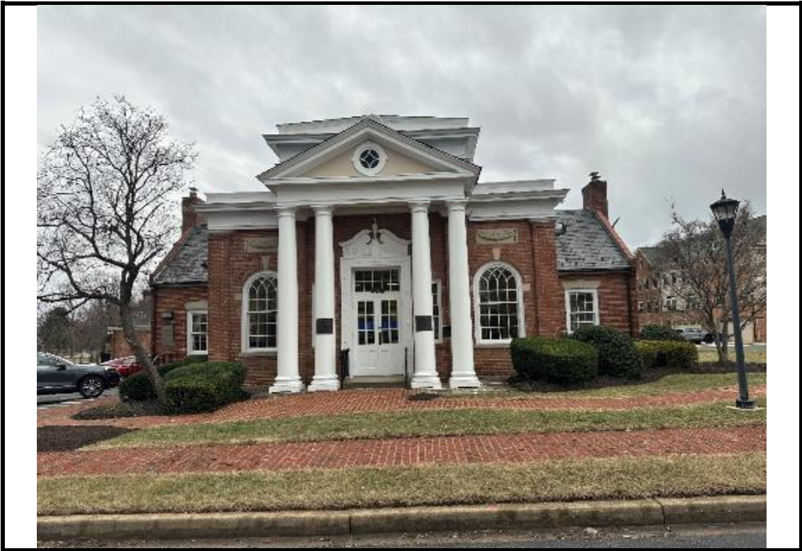
Photograph 19: General view of the building north (front) elevation.
