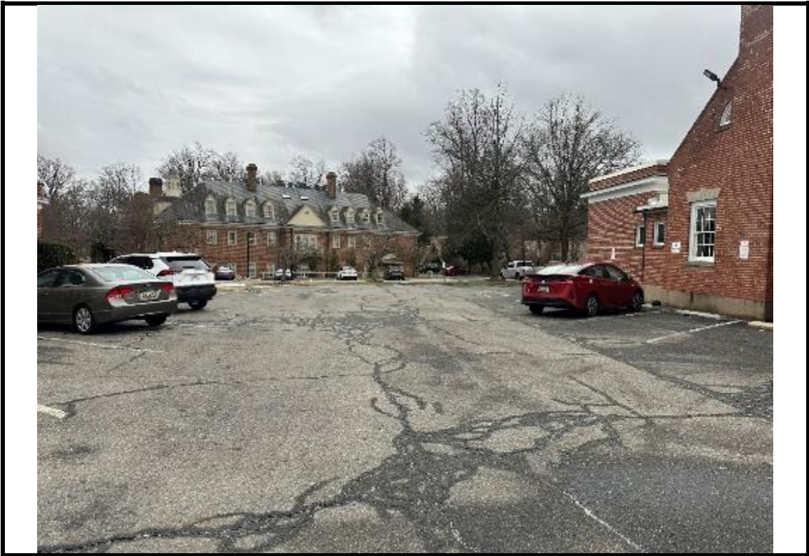
Photograph 3: General view of west parking area.
