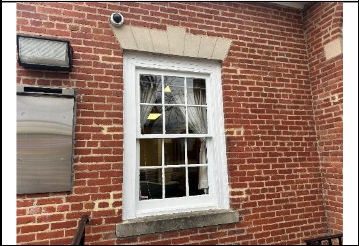
Photograph 23: Typical single-hung wood window.
