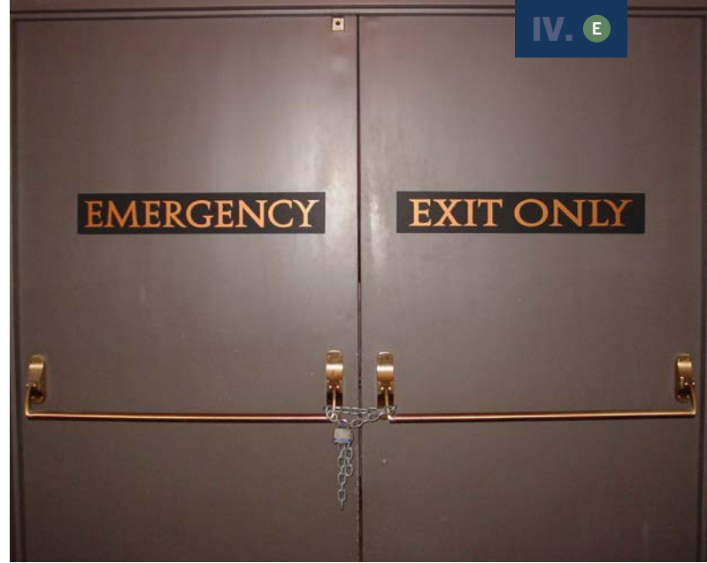
Improper locking of emergency egress. Photo Credit: Marilyn Kaplan
