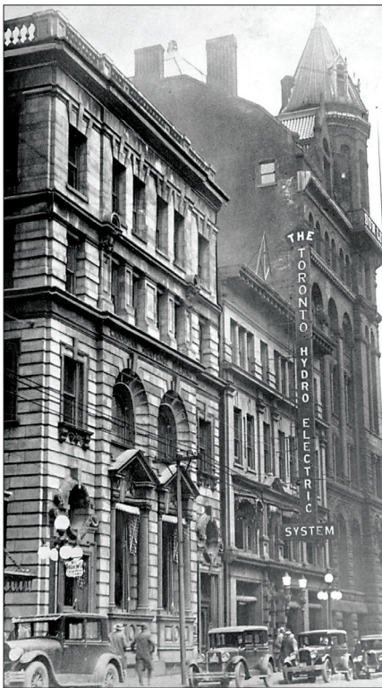
Fig. 1. Birkbeck Building, 10 Adelaide Street East, Toronto, Ontario, center, in the late 1920s. All images courtesy of Romas Bubelis/Ontario Heritage Trust.
