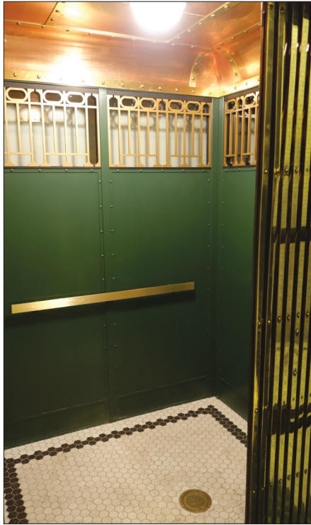
Fig. 9. Interior of the reproduction cab. Walls are post-painted, and the cove ceiling is formed from sheet-copper sections held by brass straps with rivets. The restored brass Bostwick gate appears at right.
