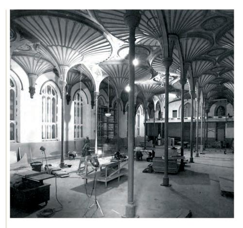
Fig. 8. A view of the chapel with the ceiling completed, December 1987. The railing of the balcony at the far end has not yet been installed.
