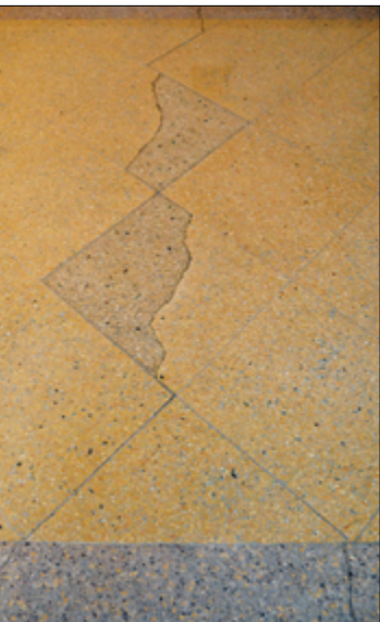
Fig. 8. Federal office building, Washington, D.C., built 1933, showing terrazzo cracking, material loss, and poorly matched infill repairs on the corridor floor. Photograph by Quinn Evans, 2021.
