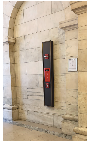
Fig. 7. Stephen A. Schwarzman Building, New York Public Library, New York, New York, completed 1911, showing the integration of fire-alarm devices in a way that respects the historic aesthetic of the space. Photograph by Michelle Dalhoff, Wiss, Janney, Elstner Associates, Inc., 2020.
