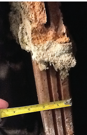
Fig. 6. Determining the fire-resistance of legacy construction materials and assemblies often requires invasive probes that should be carefully planned. In this image, the types and thickness of materials comprising an existing partition wall were determined in order to calculate its potential fire resistance. Photograph by the author, 2012.
