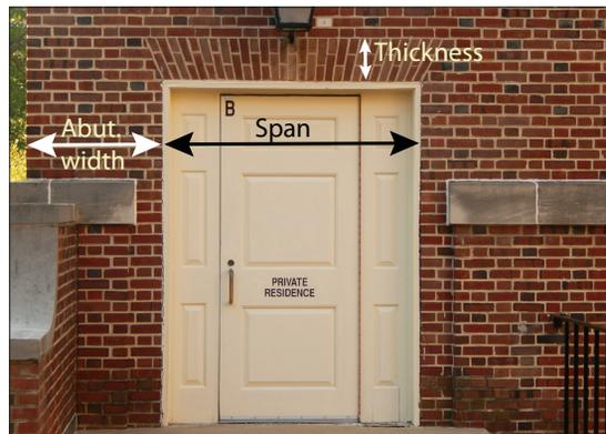
**Fig. 5.** Jordan Hall, University Park, Pennsylvania, ca. 1921, north elevation, showing a typical flat arch. The span:depth ratio is approximately 6.
