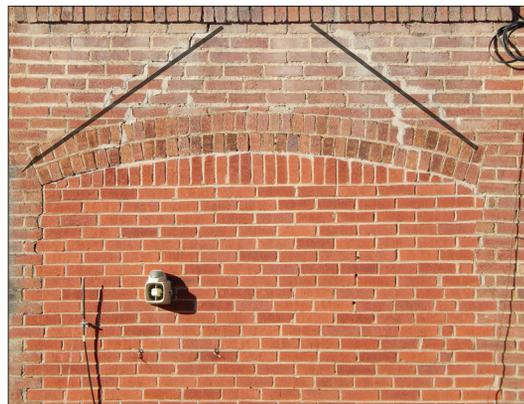
**Fig. 4.** Centre County Law Library, south elevation, showing unsymmetrical failure of a building arch.
