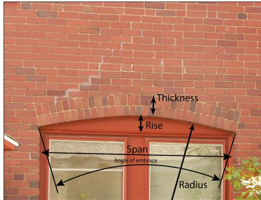
**Fig. 3.** Centre County Law Library, Bellefonte, Pennsylvania, ca. 1920, south elevation, showing abutment yielding in a flat arch. A triangular wedge of masonry has dislodged from above the arch as the arch settles.
