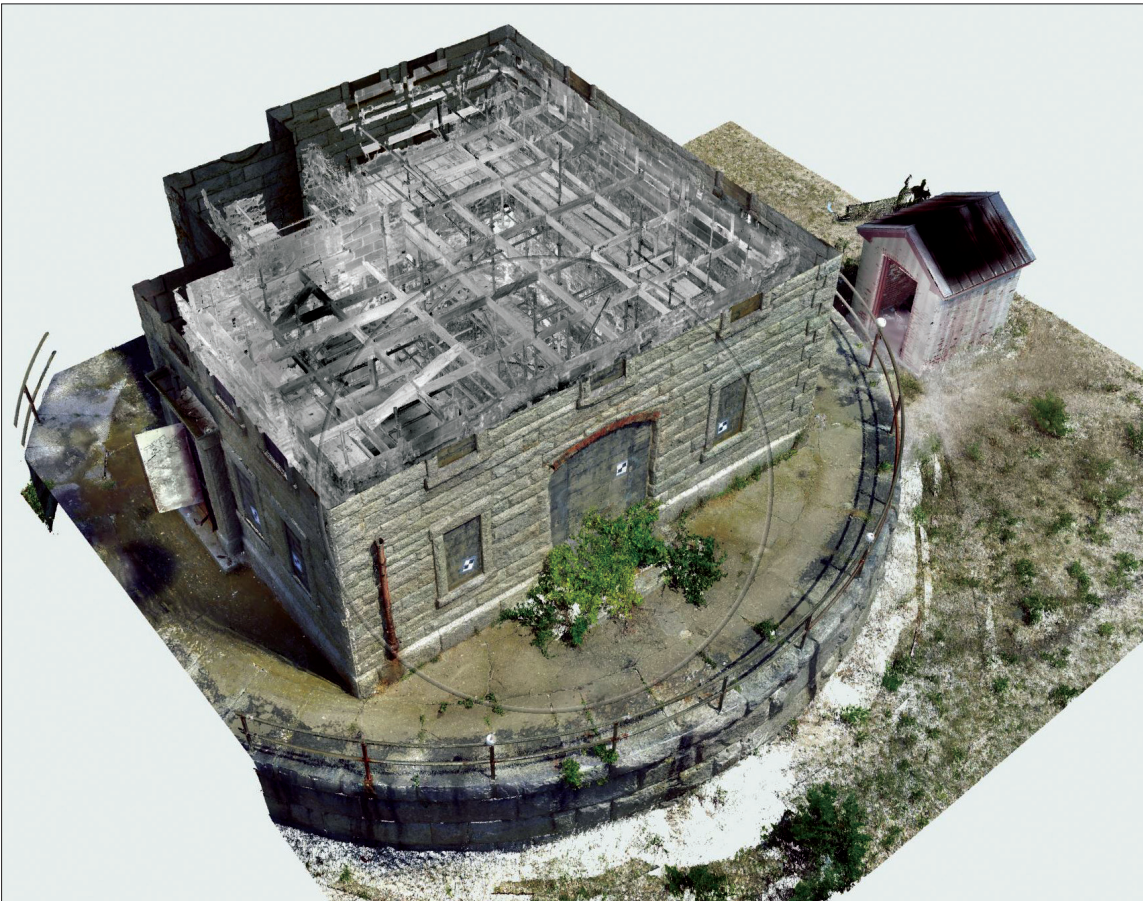
Fig. 1. Point cloud of Cedar Point Lighthouse, East Hampton, New York, built 1860. The top portion of the project point cloud is cropped to show the relationship between the interior framing and exterior walls. All figures by author.
