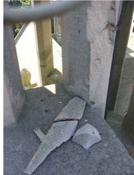
Figure 2.2: Stone spall at mechanical anchors
