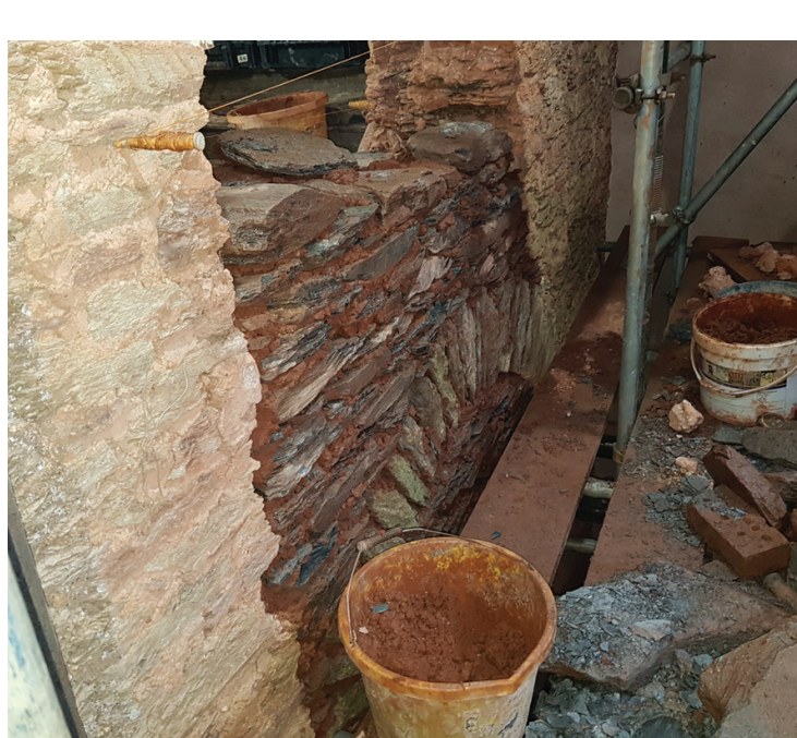
New earth mortar infill wall being built with buckets of earth mortar
