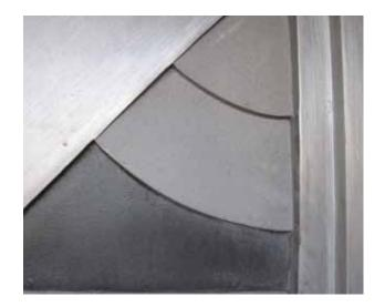
Fig. 1. Satin finish is in the upper left corner and right side. Sandblasted finish is on the upper right and middle. A replicated deplated finish is on the bottom. Samples are from a subway station in New York, New York. Images by the authors unless otherwise noted.
