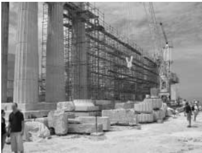
Fig. 1. The ongoing restoration of the Parthenon follows the Venice Charter and is a prime example of anastylosis. All photographs by the author unless otherwise noted.
