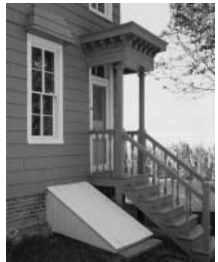
Fig. 7. Later additions to 1698 Bergen Street, such as this porch, which had been removed during the 1980s restoration in order to conform to an 1883 period restoration, were replicated in the recent restoration. Photograph courtesy of Stephen Barker.
