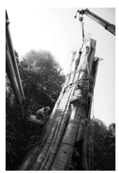
Fig. 8. The Hollow Tree supported by temporary braces, July 2008. Photograph by Harold Kalman.
