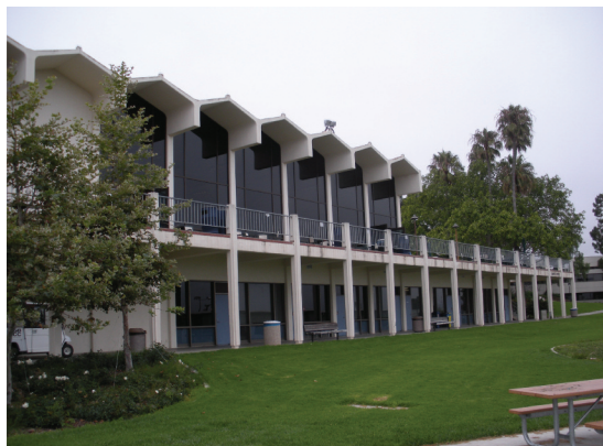
Fig. 6. College center building, west elevation, areas of testing locations for Figures 7-9.
