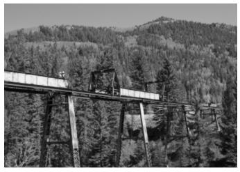
Fig. 7. A temporary gantry was used by the contractor for removing girder segments and installing new girder segments. The gantry rolls on a temporary beam that also served to provide longitudinal bracing for the structure during construction. Photograph by Roger Hogan for CTSRR.
