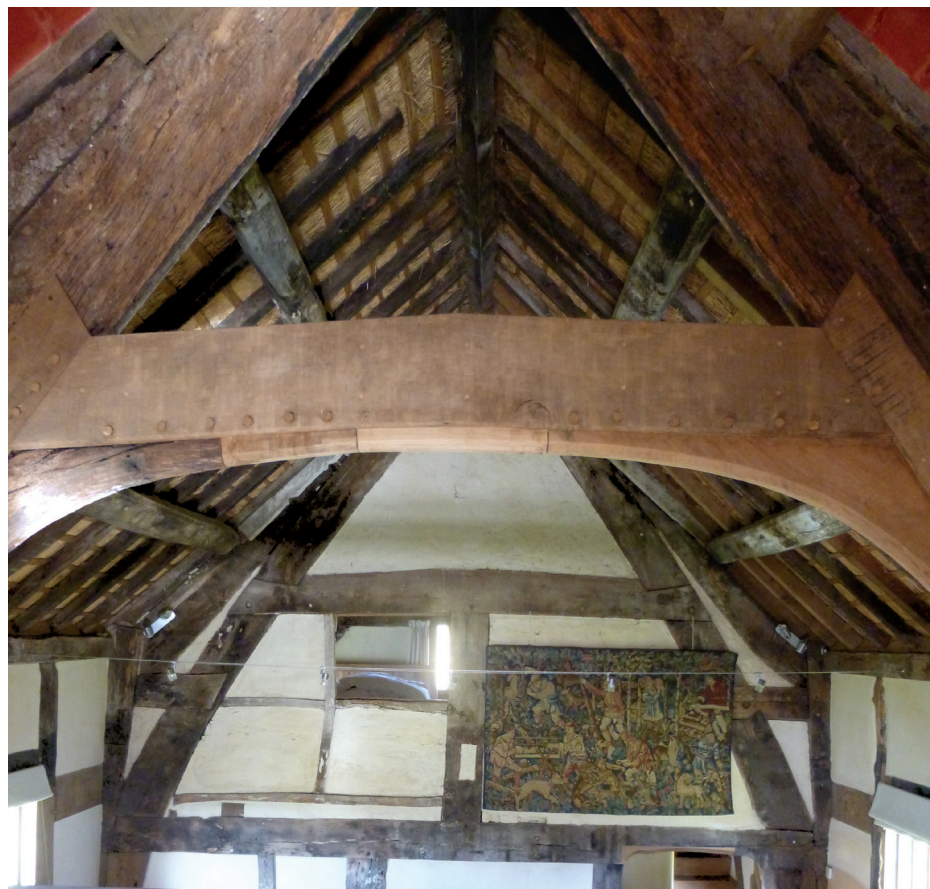
Fig. 10. Hacton Cruck Hall, interior view of central hall with bedroom beyond showing unlined thatch roof, 2015.
